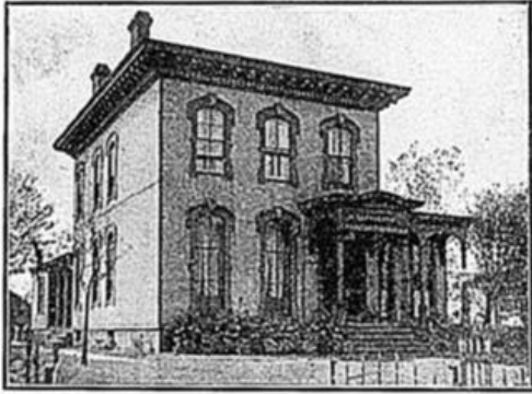
CLEVELAND CHRISTIAN ORPHANAGE. Main Building.
