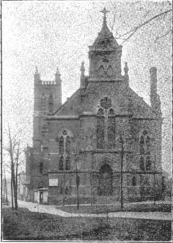
FRANKLIN CIRCLE CHURCH, Cleveland, Ohio.
