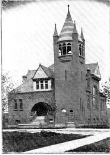
CHURCH AT BOWMANVILLE, ONTARIO
